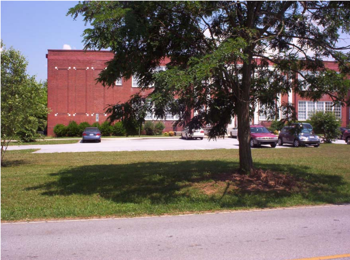
Looking West into Parkside Commons Apartments across E Blue Ridge Rd.
