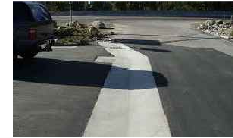
ILLUSTRATIVE IMAGE: SWALE WITH CONCRETE CHANNEL, FINAL DESIGN TO BE DETERMINED IN FIELD
