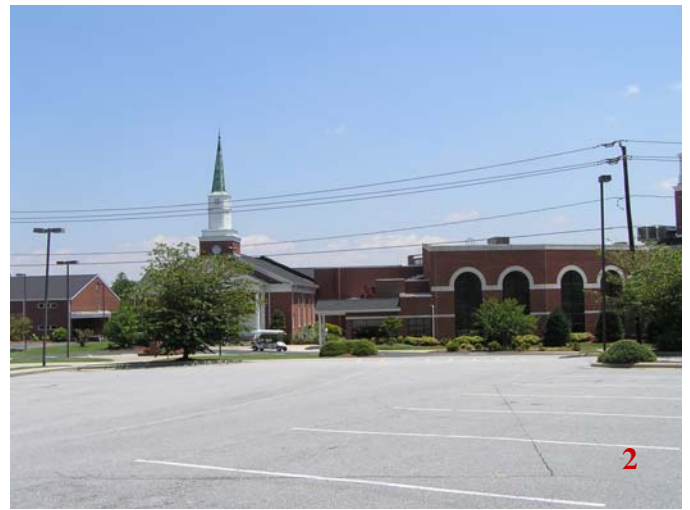
View of parking lot looking east.
