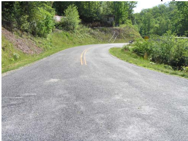
Picture of West Rock Creek Road taken from project site.
