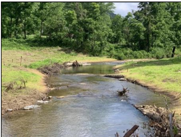
Reedy Patch Creek instream structures looking upstream, July 2020
