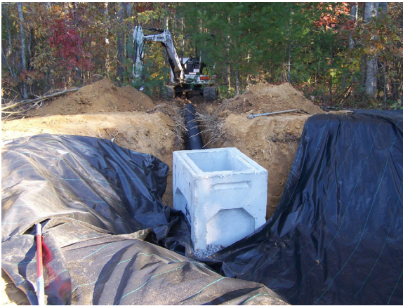
Figure 8-7. Bioretention during construction (courtesy of David Tuch, Equinox Environmental)
