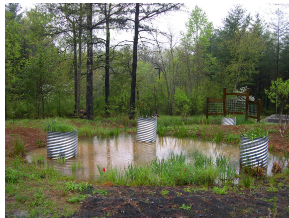
Figure 8-24. Wetland pools at the Operations Center shortly after installation
