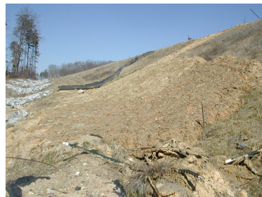
Figure 6-4. Dredged sediment dumped next to the sediment trap with no vegetation or cover
