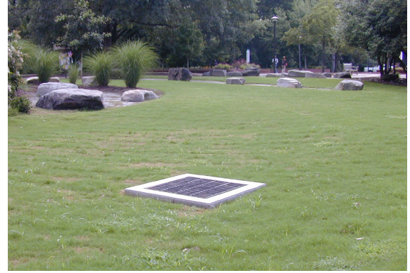
Figure 4-3. A grassed cell on the North Carolina State University campus in Raleigh, North Carolina
