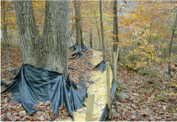
Figure 6-2. Temporary level spreader installed downstream of sediment basin in buffer
