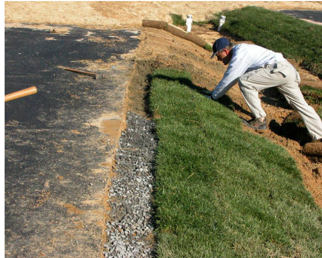
Figure 4-16. Installing a gravel verge and sod stabilizes the perimeter of bioretention cells and is highly recommended. The resulting filter strip shown here is nominally 5 feet wide.
