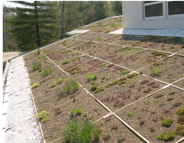
Figure 4-24. North Carolina Arboretum green roof
