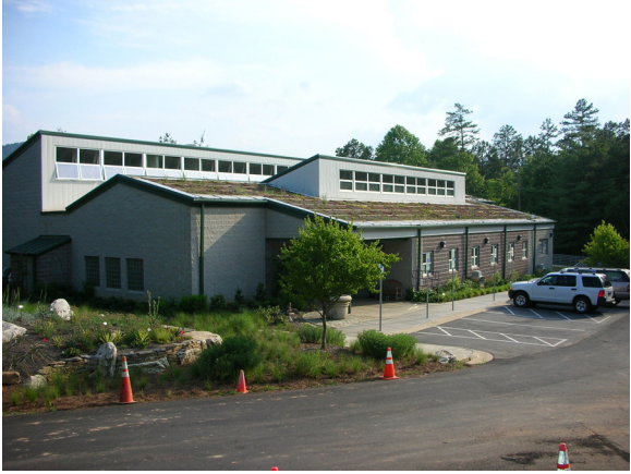
Figure 8-21. Operations Center at the North Carolina Arboretum during the retrofitting process
