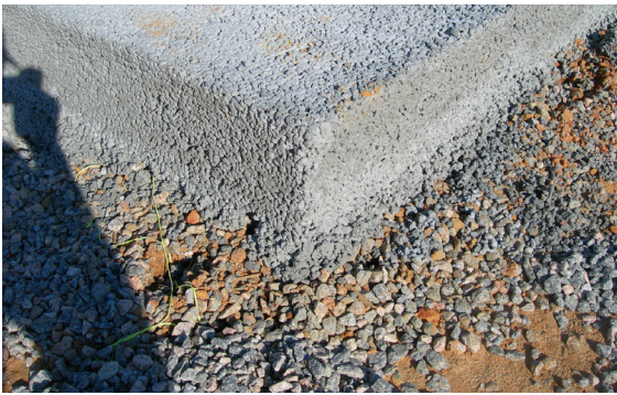
Figure 4-4. Pervious concrete in Nashville, North Carolina
