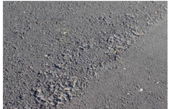
Figure 4-5. Pervious asphalt in Raleigh, North Carolina
