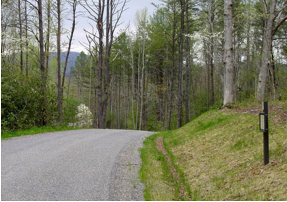
Figure 8-6. Roadside grass swales (courtesy of David Tuch, Equinox Environmental)
