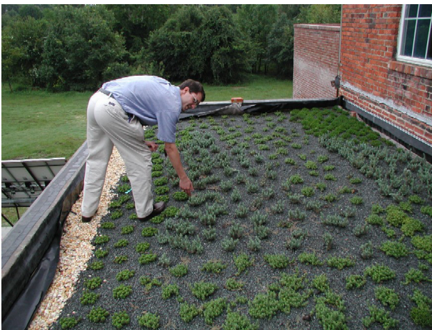
Figure 4-11. Succulent (sedum) vegetated green roof in Kinston, North Carolina
