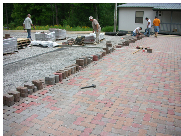
Figure 8-25. Installing the permeable parking lot at the Operations Center
