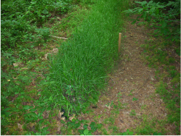
Figure 8-26. Level spreader at the Operations Center
