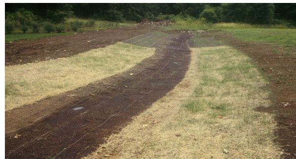
Figure 4-22. Turf reinforcement matting installed in a swale in Durham, North Carolina
