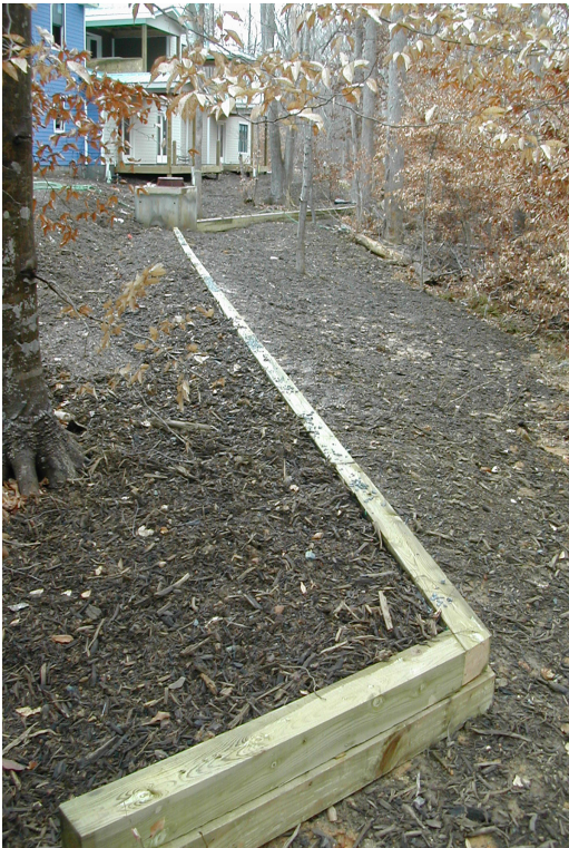
Figure 6-5. Level spreader in a preserved wooded buffer downstream of an LID project
