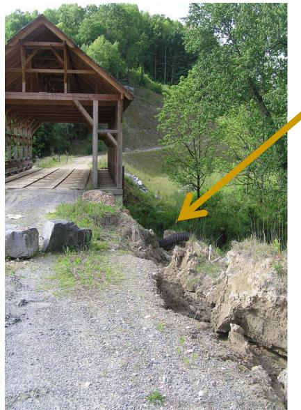
Significant Erosion Around Bridge Support
