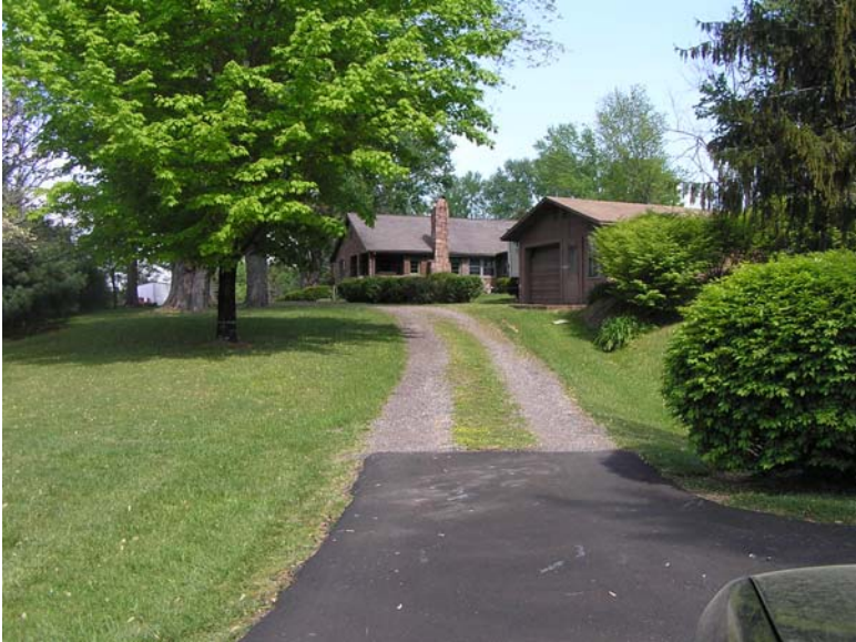
Single-family residence on Subject Area.
