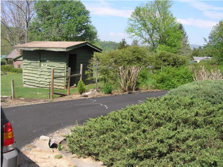
View of rear yard
