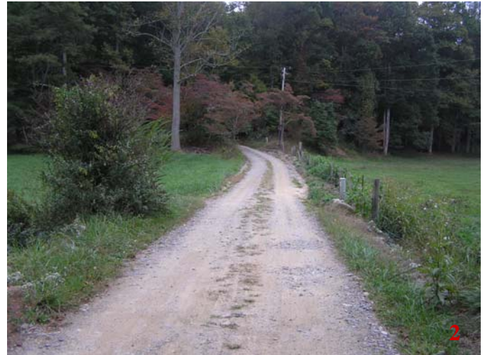
2. View of a portion of Old Pace Farm Lane, which is adjacent to, and partially located on the Project Site and remainder tracts. Old Pace Farm Lane is one (1) lane (10 to 11 feet in width), is not constructed of adequate gravel/asphalt; and lacks shoulders, ditches and turnarounds.
