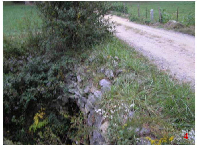
4. View of the culvert along Old Pace Farm Lane.
