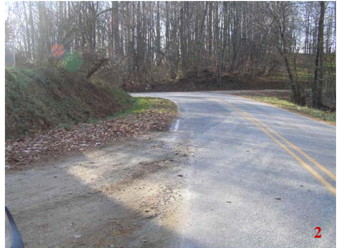
2. View of from Clark Gap Drive cut onto Hutch Mountain Road looking west into curve. The applicant intends to realign the road due to the existing angle of intersection and low visibility.
