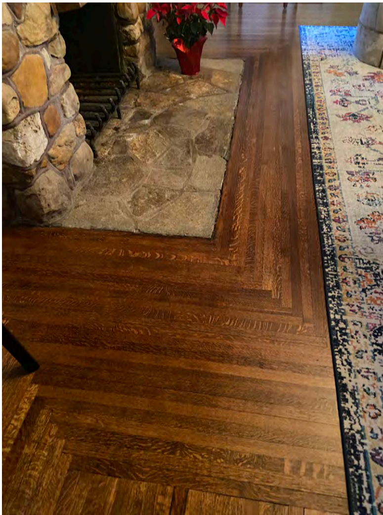
Picture Framing in Wood Floors
