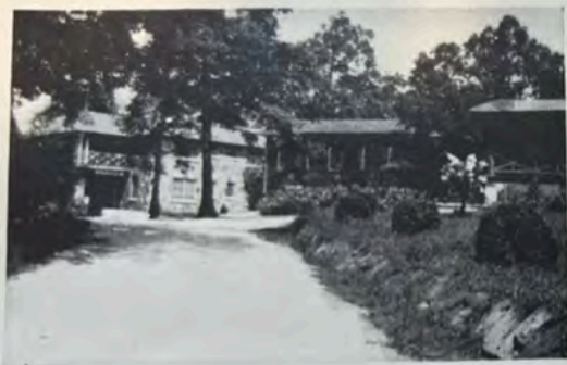
Guest House and Dining Hall of Lodge
