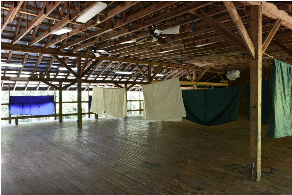
New Lodge (#24), interior, view to southeast
