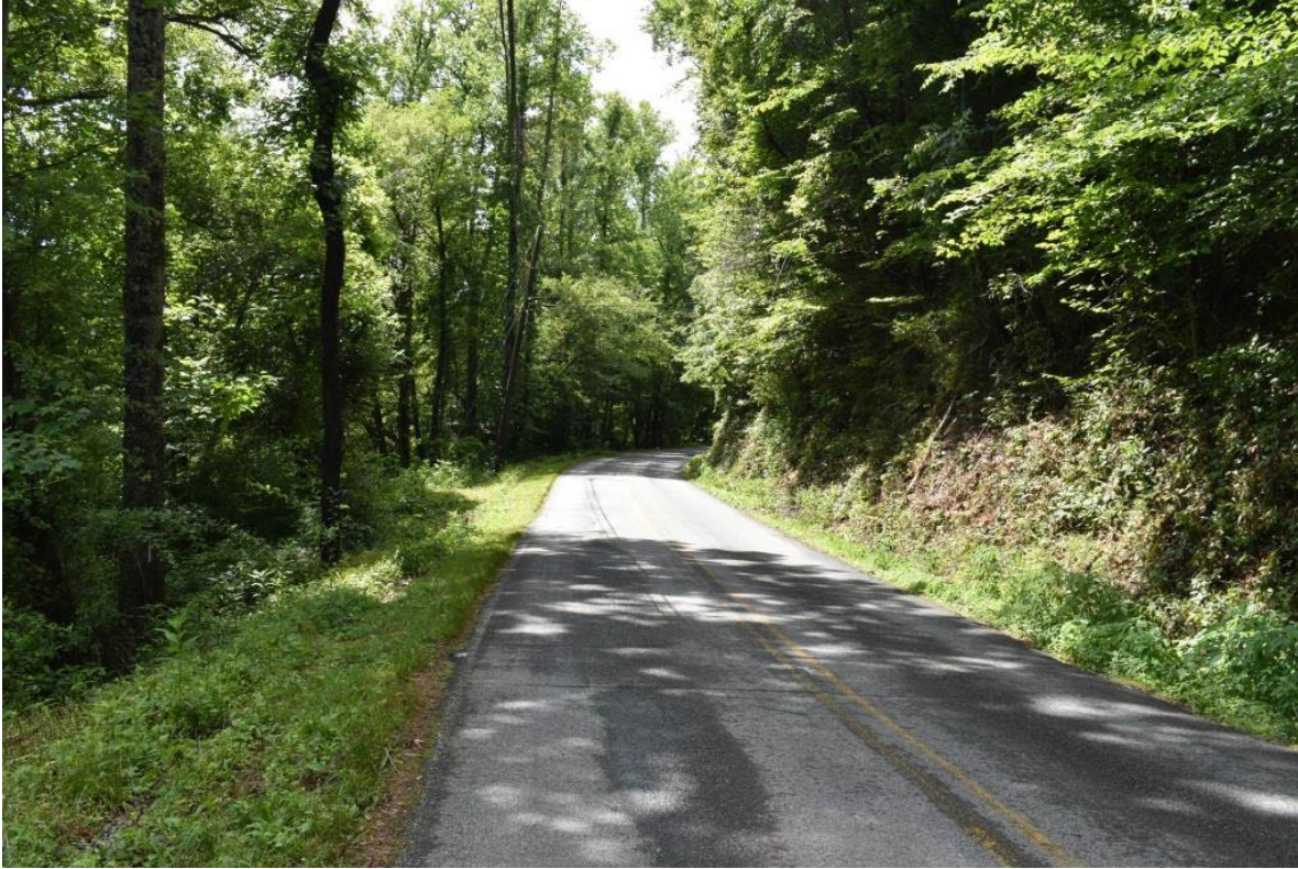
SR 1534 (Hart Road), view to southeast
