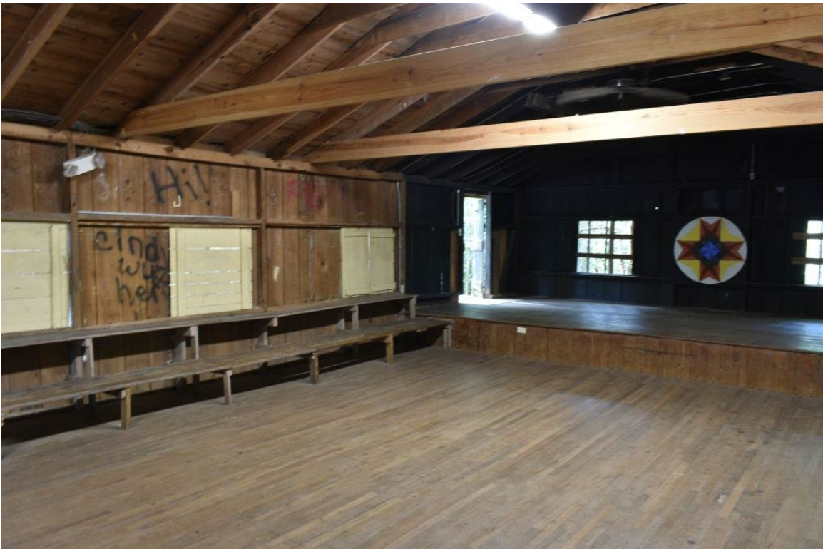
Old Lodge (#2), interior, oblique view to north end
