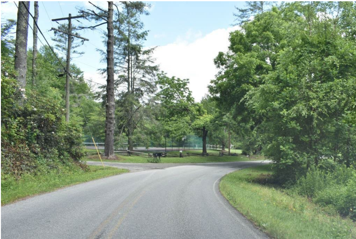
SR 1534 (Hart Road) at intersection with Eagles Nest Lane, view to northwest
