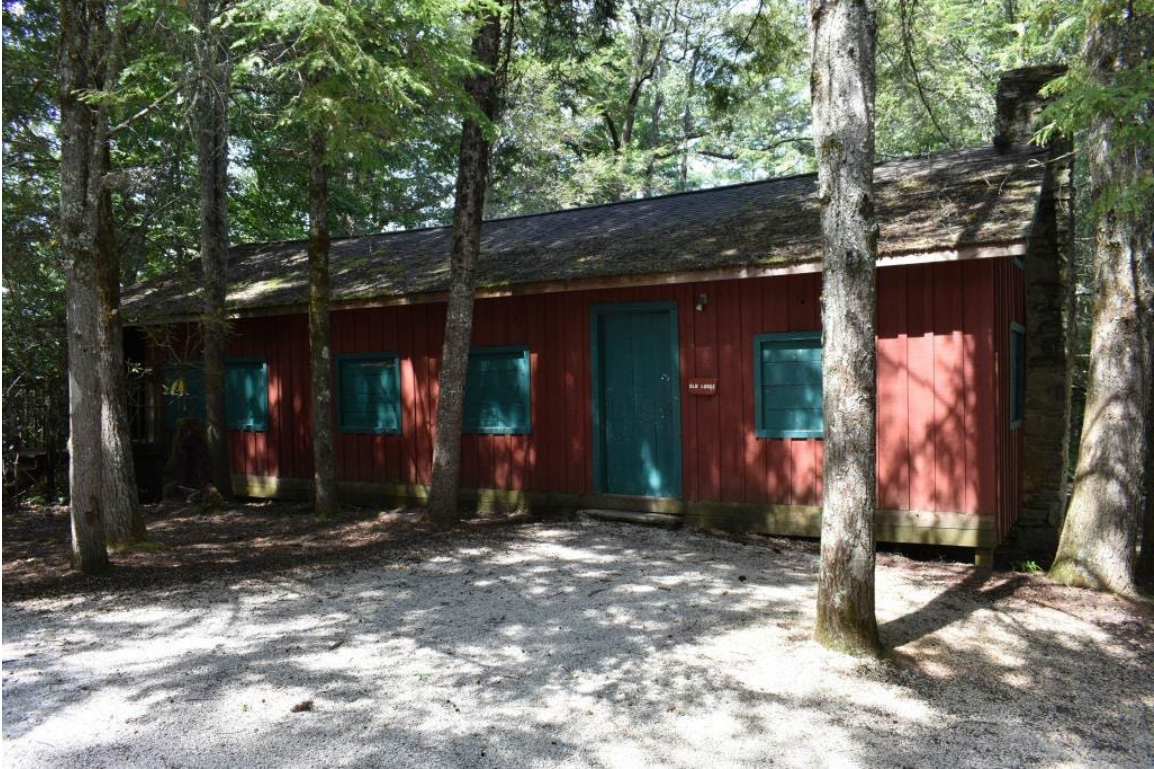
Old Lodge (#2), southwest elevation, view to north
