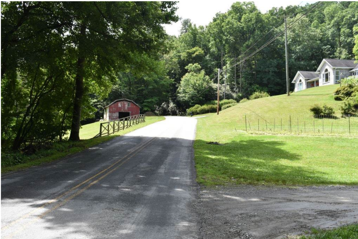
Project end, SR 1534 (Hart Road), view to south
