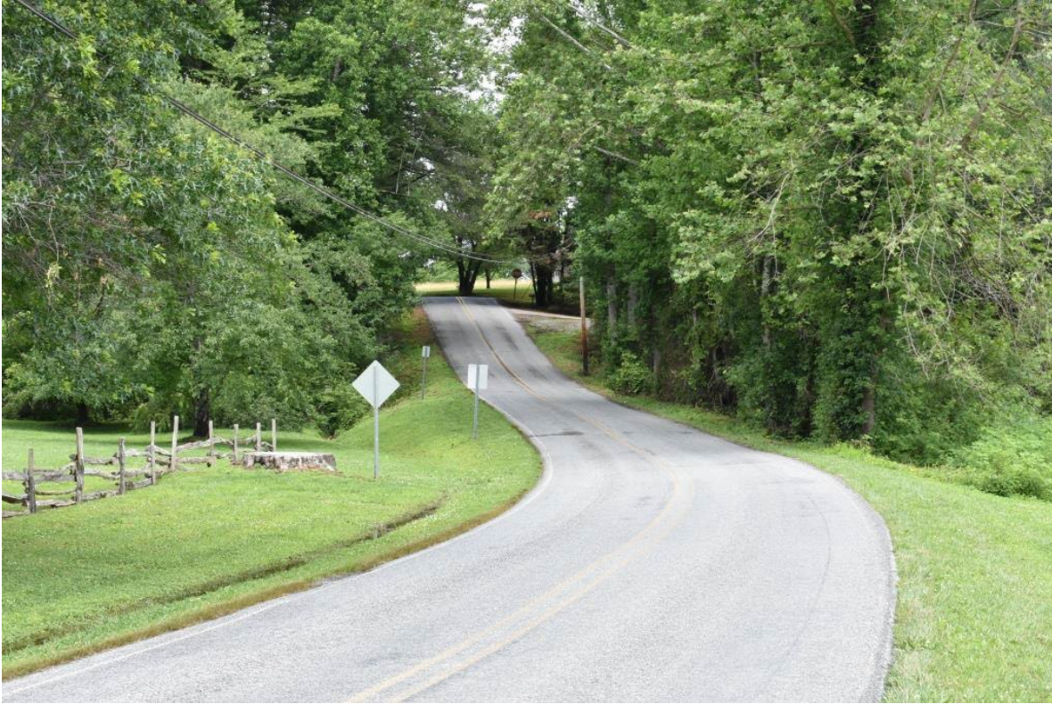
SR 1534 (Hart Road), view to northwest through Eagle's Nest Foundation property
