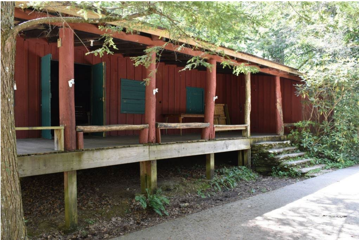
Old Lodge (#2), northeast elevation, oblique view to west
