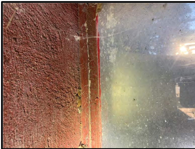
Photo No. 2 – Homogeneous Area A-11 Metal Window Interior Glazing
