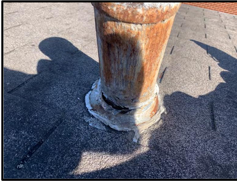
Photo No. 1 – Homogeneous Area B-13 Black Flashing Material
