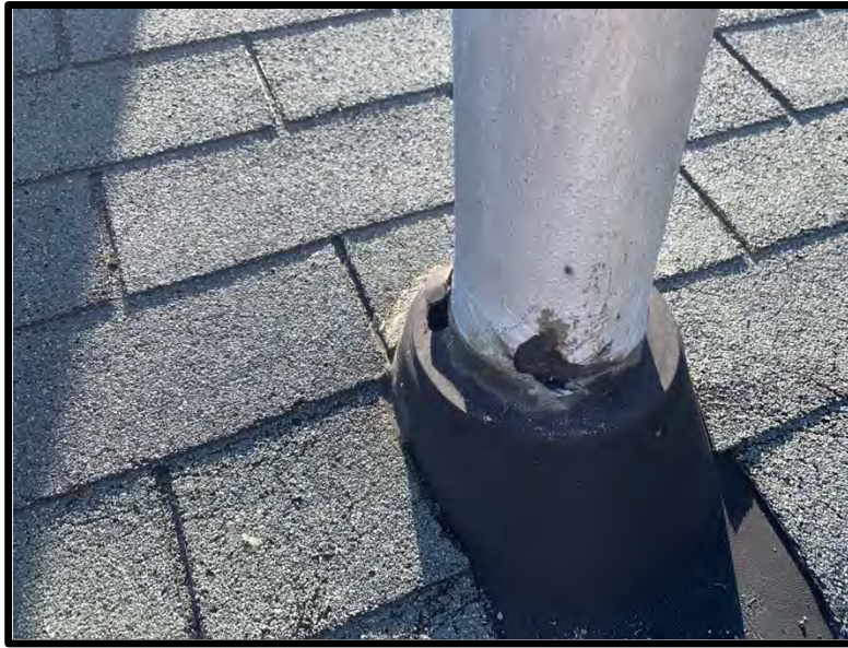
Photo No. 3 – Homogeneous Area A-14 Silver Painted Black Flashing Material
