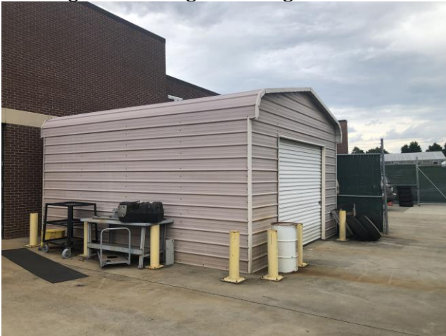
Existing Auto Storage Building
