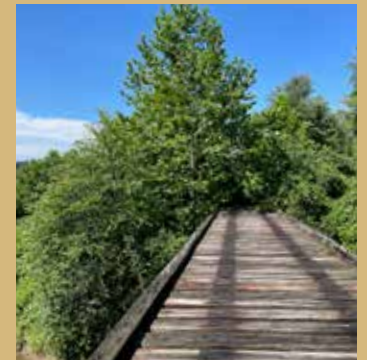
Rail bridge over the French Broad River.
