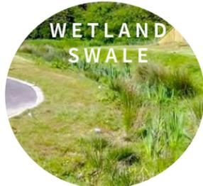
Swales are crucial to greenways in flood-prone areas and can be either by a grass swale, or a wetland swale if water table levels are high. Dry swales are typically planted with grasses and should not be mowed to allow for maximum infiltration of water. The wetland swale is appropriate where the water table is high or stormwater collects for longer periods of time.
