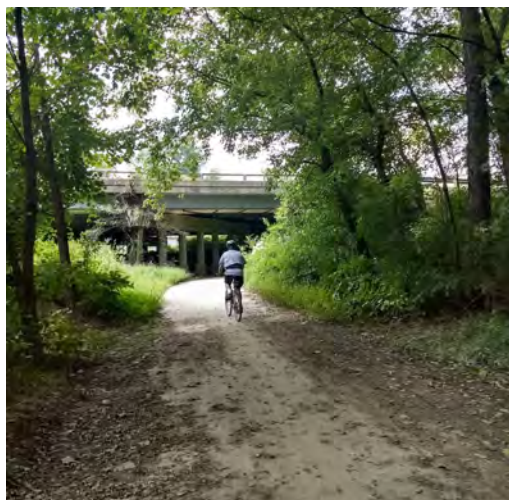
Debris caused by receded flood waters on trail before Hwy 64 underpass
