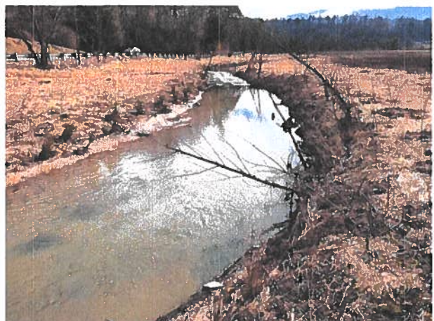
After Construction, January, 2021
