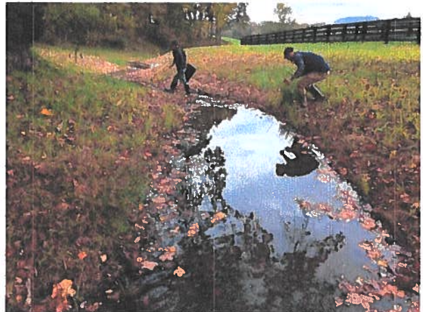
After Construction, October, 2020
