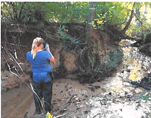
Before Construction, November, 2017
