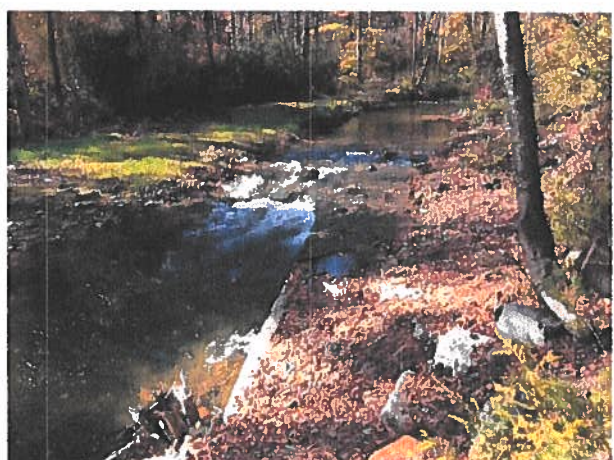
After Construction, October, 2020
