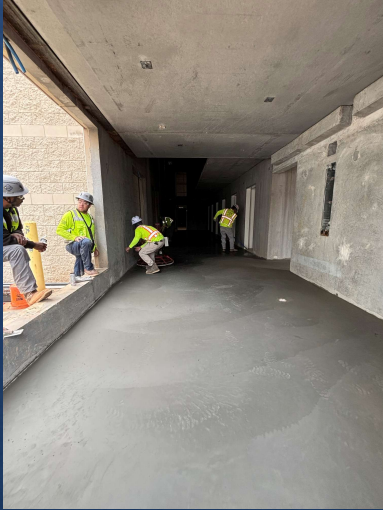
Pouring Slab in Women's Expansion
