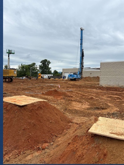
Aggregate Piers for New Sally Port
