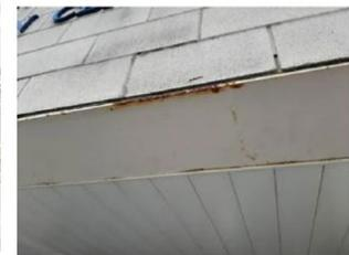
Figure 2 – Example of rust at lintel
