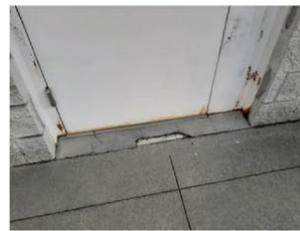
Figure 7– Rust at exterior doors and frames.
