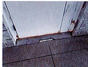
Figure 7 – Rust at exterior doors and frames.
