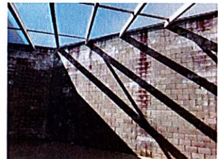
Figure 11 – Mold and efflorescence at minimum housing recreation yard
