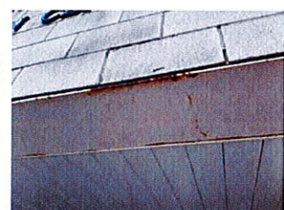
Figure 2 – Example of rust at intel
