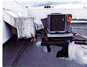
Figure 3 – Roof at support area-Equipment drainage
