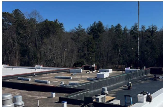
HVAC Project at Atkinson Elementary School
