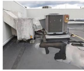
Figure 3 – Roof at support area-Equipment drainage
