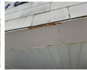
Figure 2 – Example of rust on Intel
