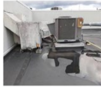
Figure 3 - Roof at support area Equipment drainage
