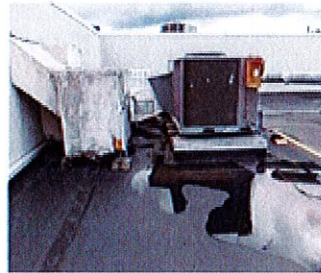
Figure 1 - Roof of support area Equipment drainage
