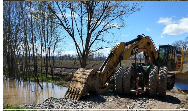
Restoration: Grading and Construction
