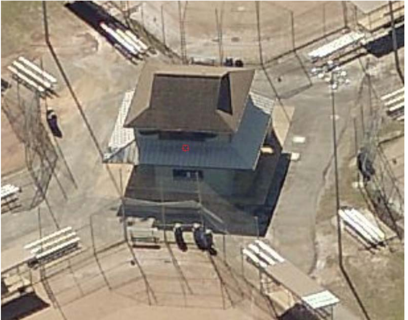
3. Etowah Park Existing Facility Building
