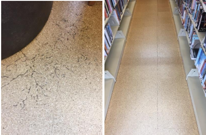
FY20-21 / Replace cork flooring / Impact: $25,000
