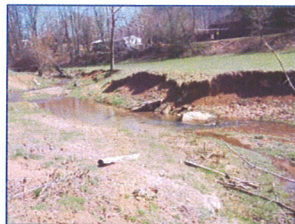
Severe Bank Erosion along Reedypatch Creek
