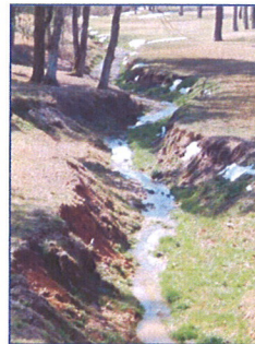
Erosion along Devils Fork
