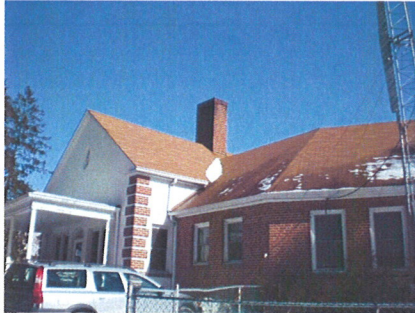
1-L-- Structural repairs and new metal roof-- $50,000.00
