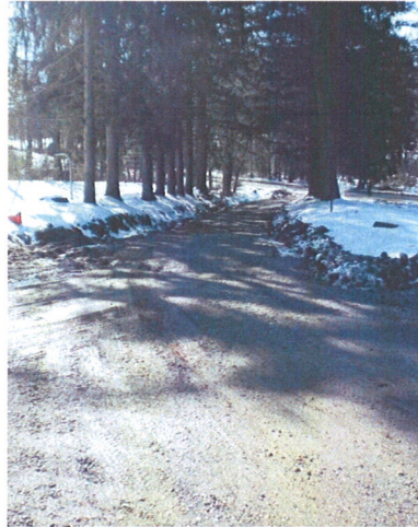
2-D Paving and Drainage Improvements at Stoney Mountain Activity Center --$50,000.00
