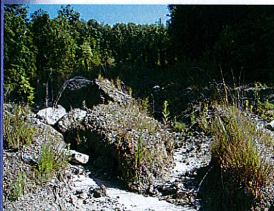
Site Prior to Work (July 2013)
