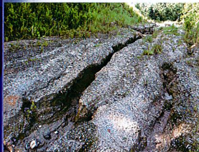
Site Prior to Work (July 2013)
