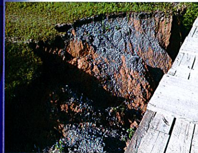
Site Prior to Work (July 2013)
