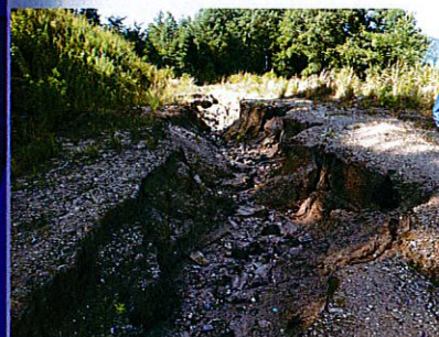
Site Prior to Work (July 2013)
