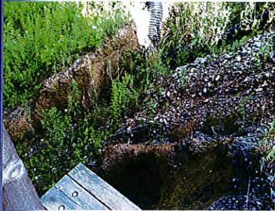
Site Prior to Work (July 2013)
