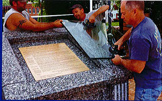
Each of the six documents will be original size on .25" etched bronze, weighing over 60 lbs., and mounted 3" under a 1/4" sheet of laminated viewing glass.
