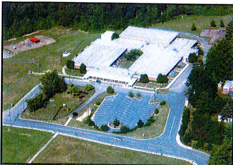
aerial view of HENDERSONVILLE ELEMENTARY
