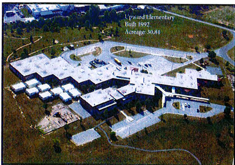
aerial view of UPWARD ELEMENTARY
