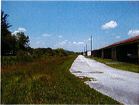
Close proximity to hangers
