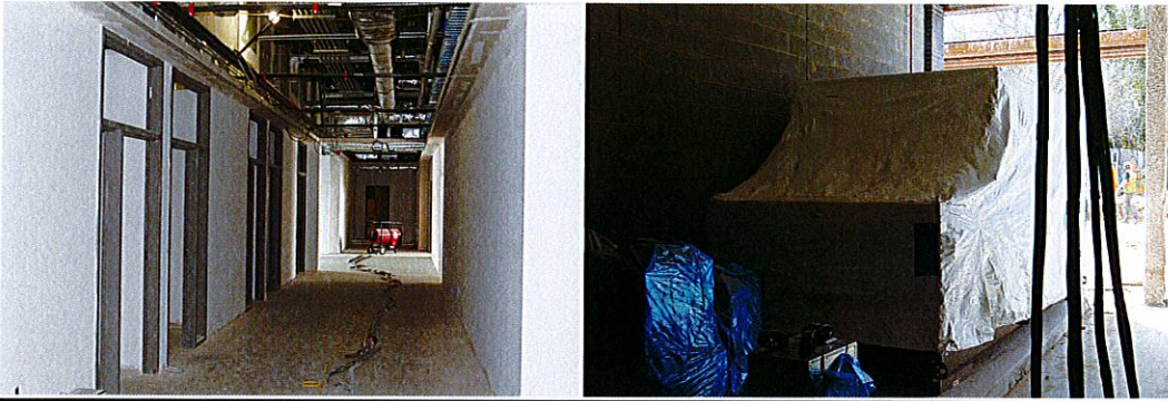
Air handling unit
