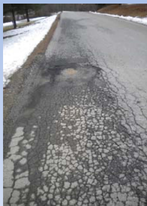
1-A Full depth patching and resurfacing--$120,000.00
