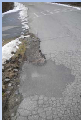
1-A Full depth patching and resurfacing--$120,000.00
